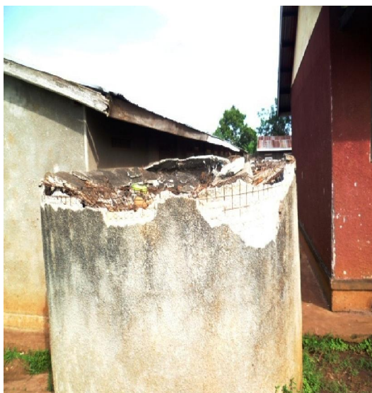
The old broken concrete water tank
